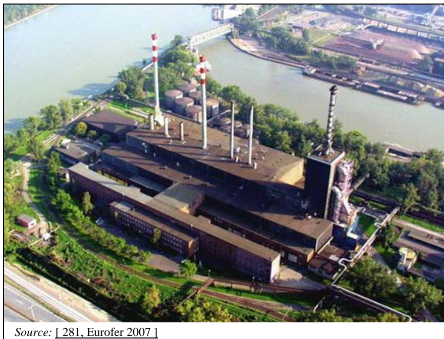
Figure 2.6: View of a power plant in an integrated steelworks
