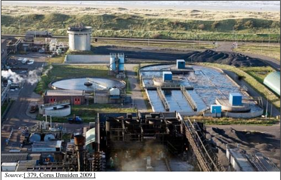
Figure 5.24: Aerial view of the biological waste water treatment plant at Corus, IJmuiden, the Netherlands
